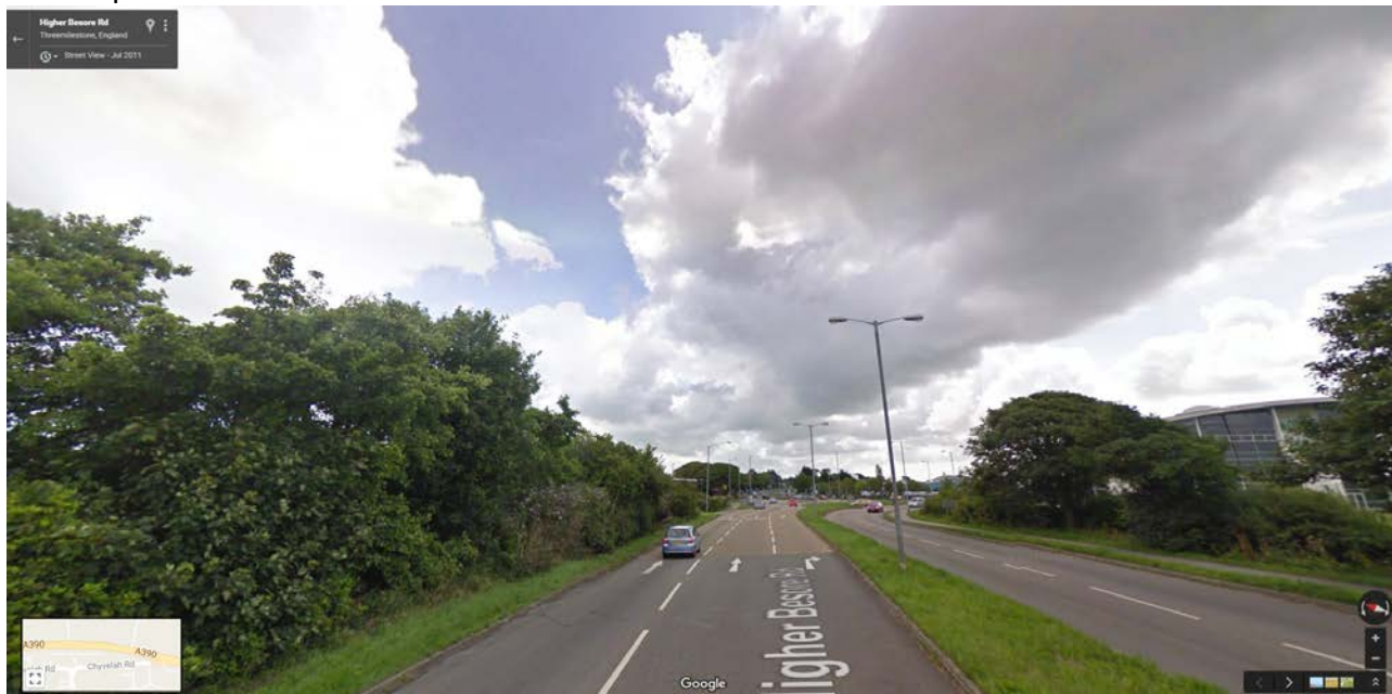
Figure 28: The A390 near Threemilestone
